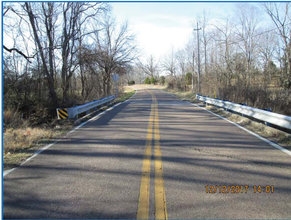
Looking west across bridge standing near east end of bridge
