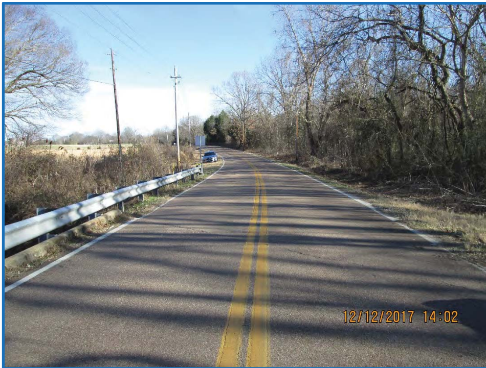
Looking east standing near middle of bridge
