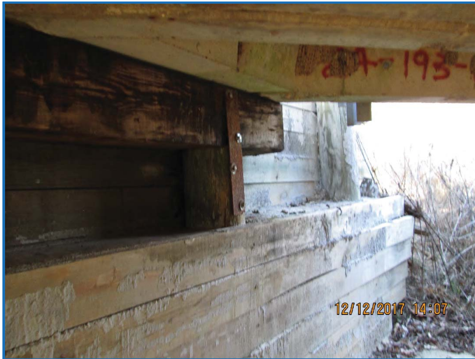
Looking at west abutment standing under bridge
