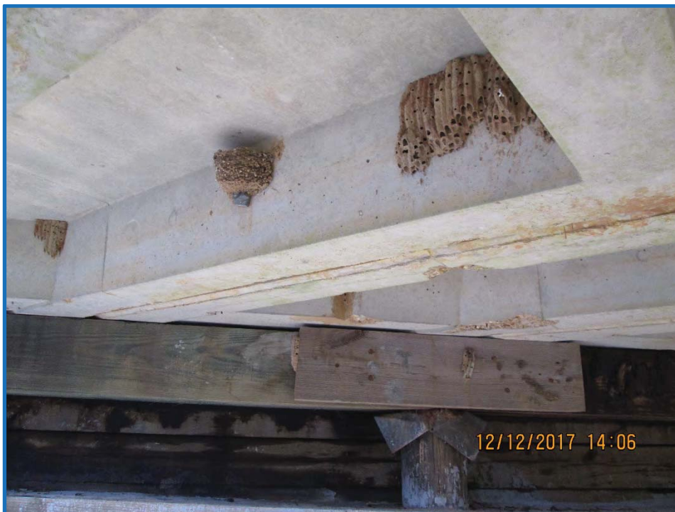
Looking under bridge deck
