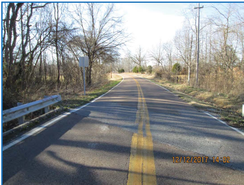
Looking west standing near middle of bridge
