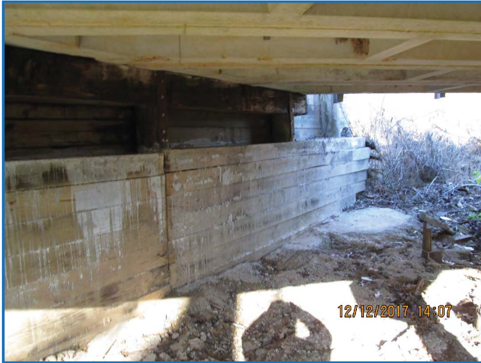
Looking at west abutment standing under bridge
