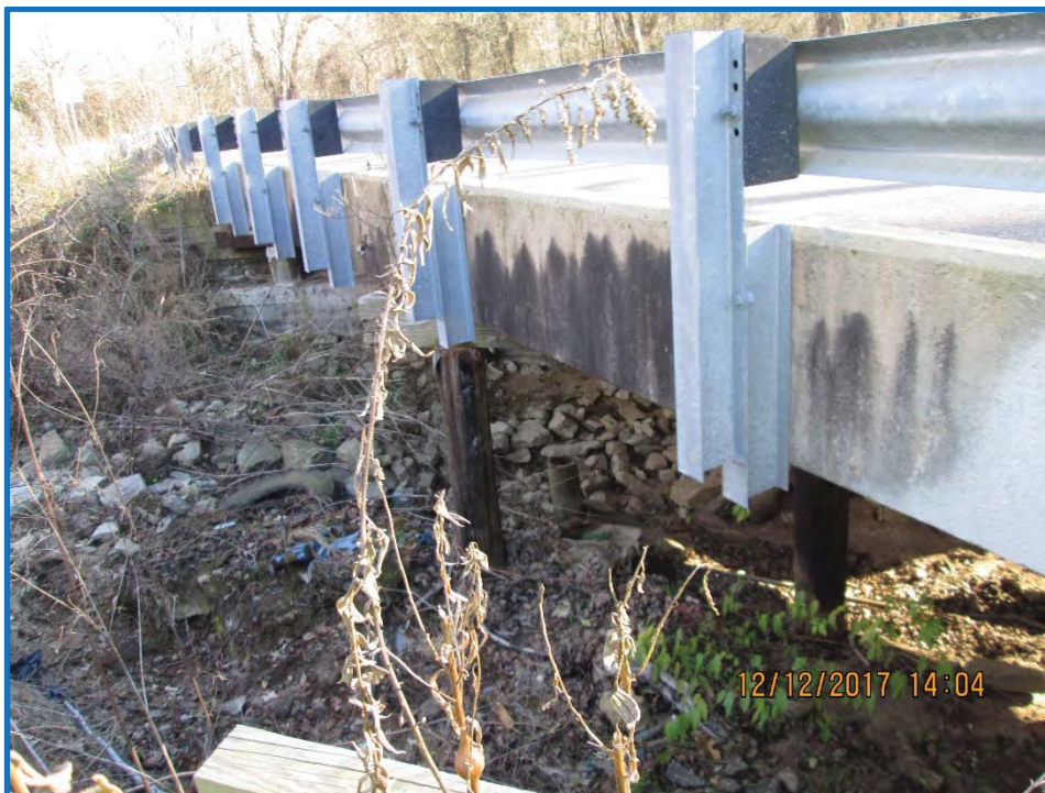
Looking at upstream side standing off NW corner of bridge
